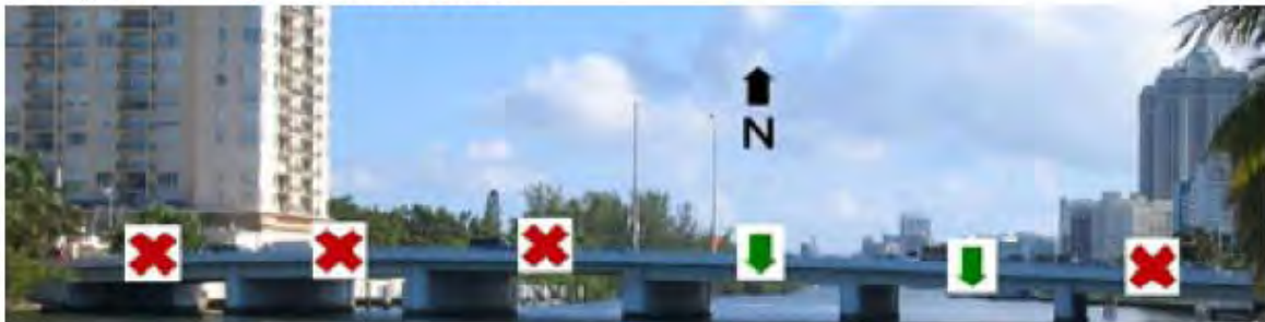
Bridge at 41 st street north bound
